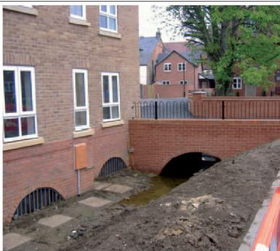
Fig 9 Flood protection with boundary wall and draining
