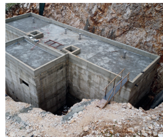
'ROCK SOLID' - the new 400 m 3 water reservoir has literally been built into rock.
