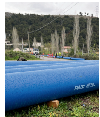
Huge pipes with a diameter of 500 mm diameter are now assuring 24/7 water supply for Shengjin.
