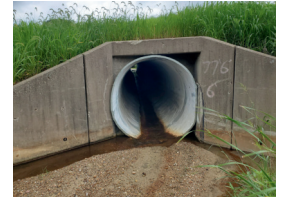
Stormwater culvert - catching and draining stormwater
