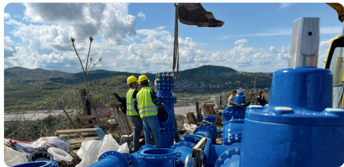
New main distribution pipes are installed.
