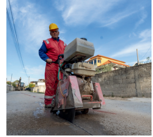
Cutting asphalt for preparing installation of network.
