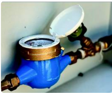
Individual water meters - key for fair, transparent and just invoicing of water consumption.
