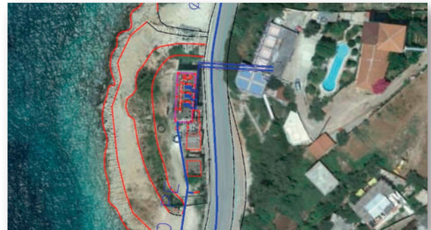
Aerial view of Pumping Station 6 - Rehabilitation of Sea Water Protection Dam
